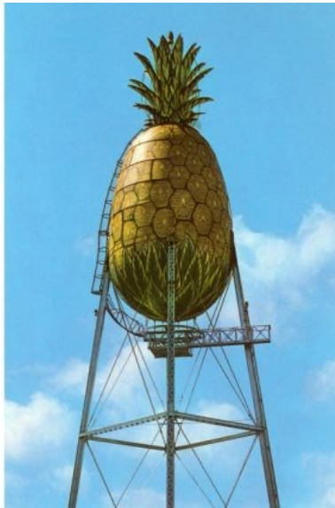
Dole Cannery Water Tower
